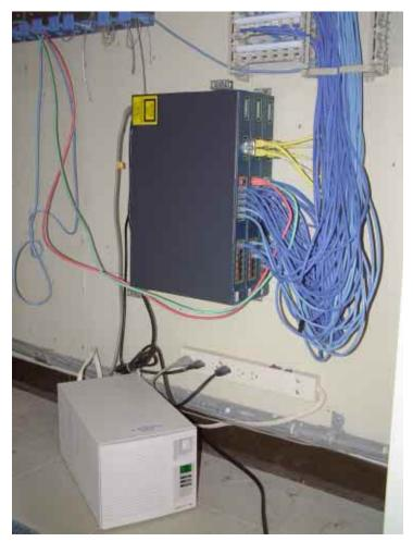
that was not happening. Upon closer examination, it turned out that the switch was not fully power cycling. Instead, it was due to more subtle power disturbances which were severe enough to reset the ports going to the desktop, thus freezing the computers.
